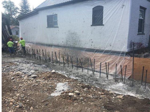
Figure 5 Micro pile retaining wall
