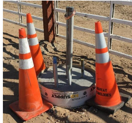
Figure 4 Light pole caisson
