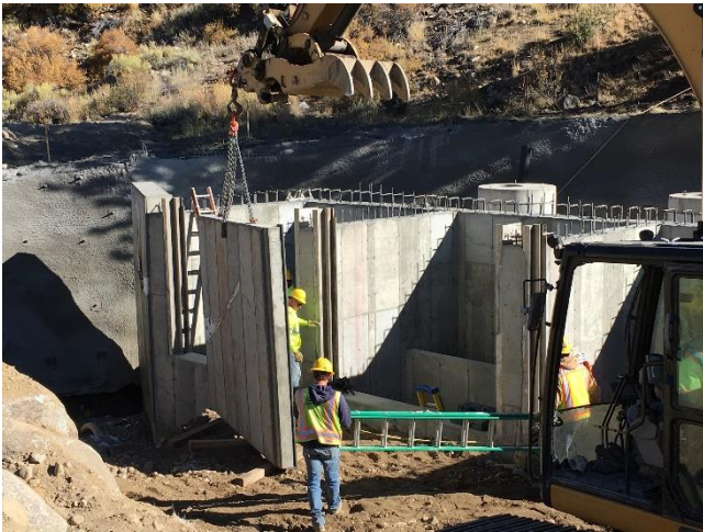
Figure 2 Water intake bulk head
