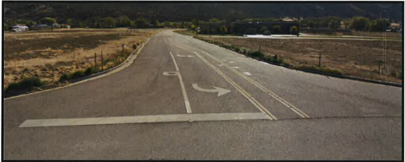
Figure 9-Vandaveer Ranch Road looking East from Highway 50
