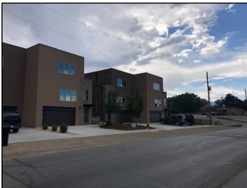
View of duplex buildings adjacent the subject property (view looking northwest)
