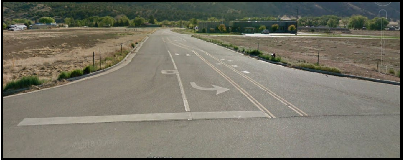
Figure 6-Vandaveer Ranch Road looking East from Highway 50
