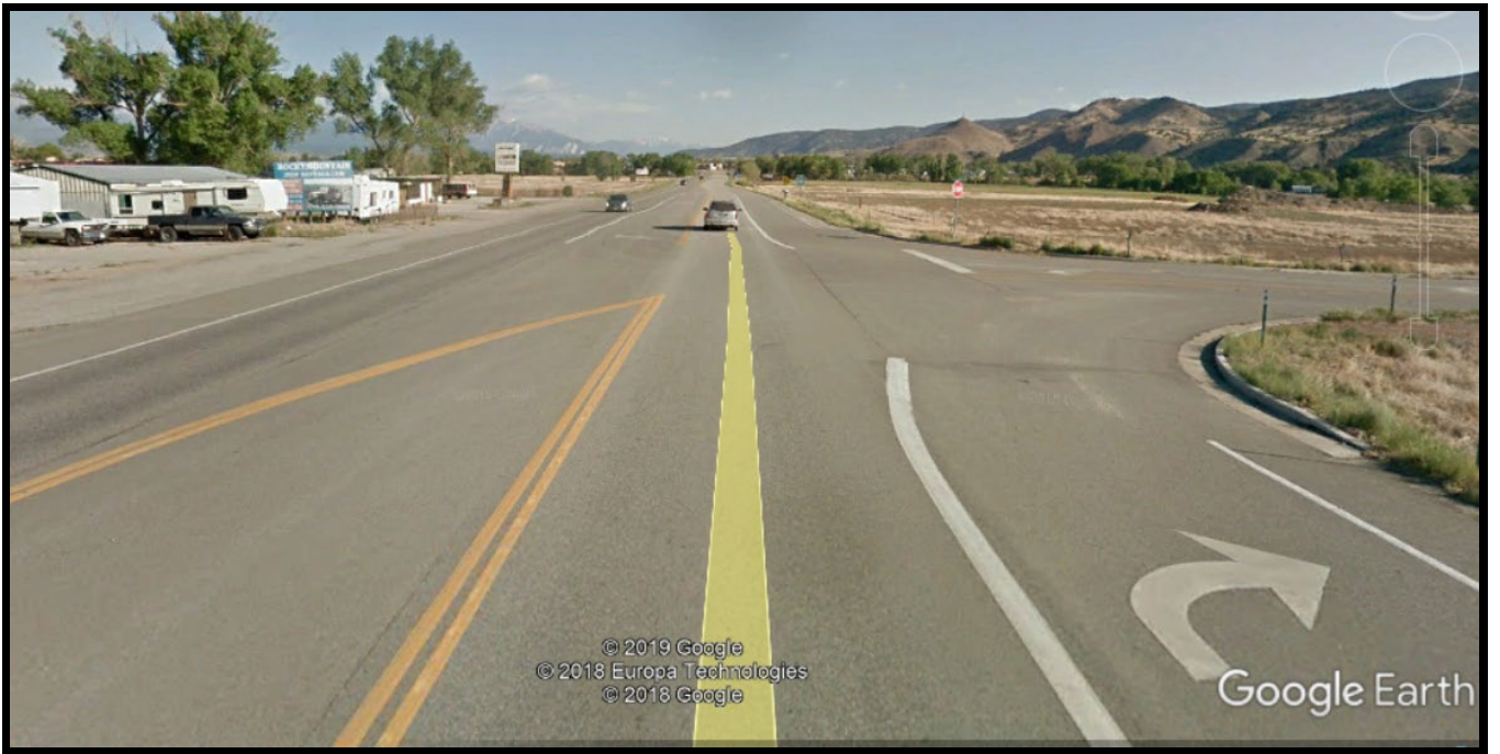
Figure 5-Highway 50 looking North West at Vandaveer Ranch Road
