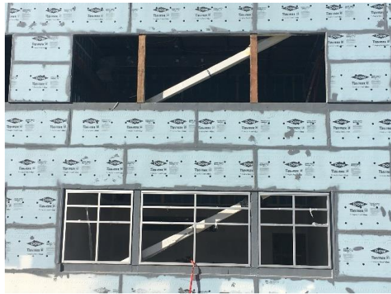
Figure 2. View from outside of classroom
