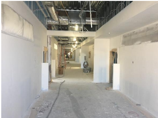
Figure 3. View of 70% completed hallway
