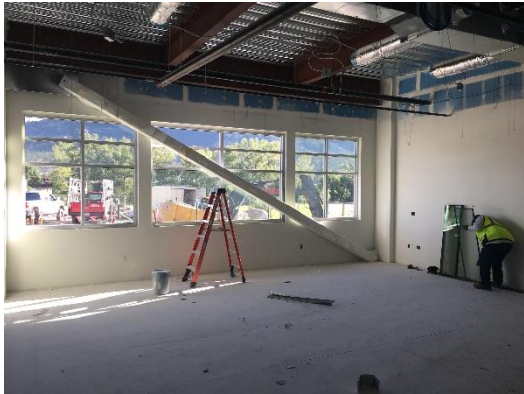
Figure 1. View from inside of classroom
