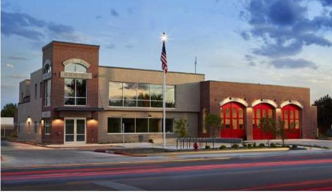
Public facing, inviting, know where entrance is, clean lines, timeless, long-lasting, set tone for future development in area
