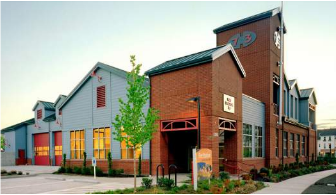
Like wrap around corner (2 faces to building)
