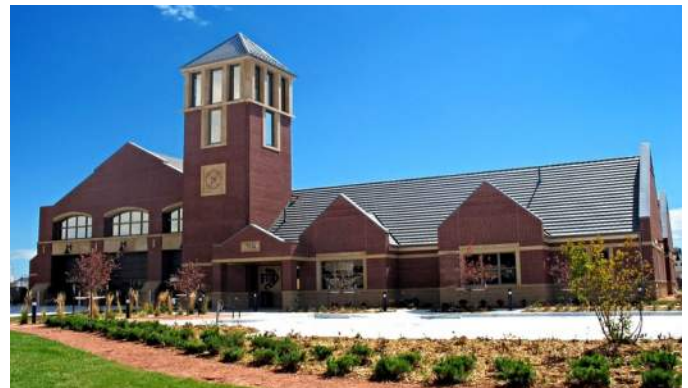
Tower is too tall
