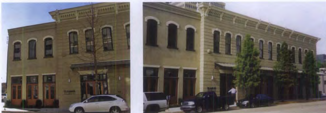
Figure 28. A small addition (left) was constructed when this 1880s train station was converted for office use. The paired doors with transoms and arched windows on the compatible addition reflect, but do not replicate, the historic building (right).
