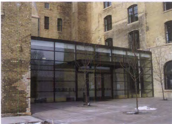
Figure 14. This glass addition was erected at the back of an 1895 former brewery during rehabilitation to provide another entrance. The addition is compatible with the plain character of this secondary elevation.
