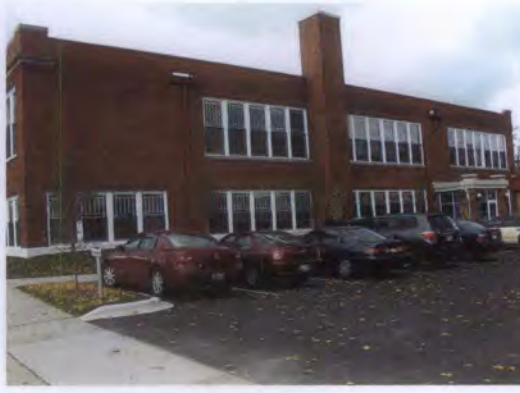
Figure 29. This simple glass and brick entrance (left) added to a secondary elevation of a 1920s school building (right) is compatible with the original structure.
