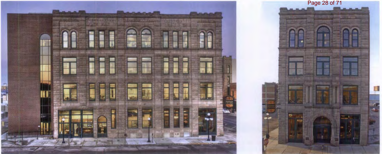
Figure 27. Although the new brick stair/elevator tower (left) is not visible from the front (right), it is on a prominent side elevation of this 1890 stone bank. The compatible addition is set back and does not compete with the historic building. Photos: Chadd Gossmann, Aurora Photography, LLC.
