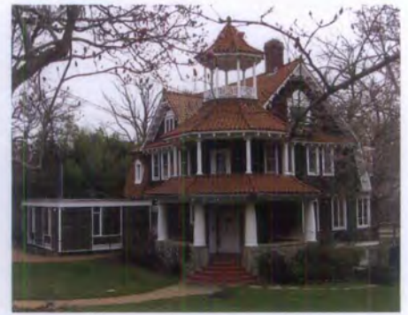
Figure 17. The small addition on the left is starkly different and it is not compatible with the eclectic, late-19th century house.
