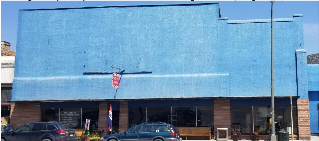
Image #2 (below) Front elevation of existing structure, August 24, 2018
