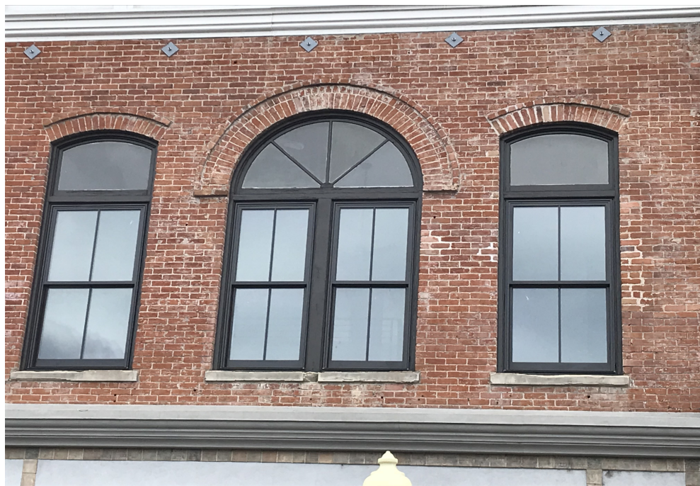
Photo 5: Talon RetroFit window insert used in the Unique Theater.
