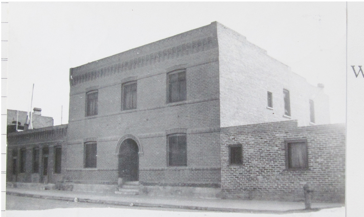
Image #2: Laura Evans Building (129 W. Sackett) before application of stucco.
