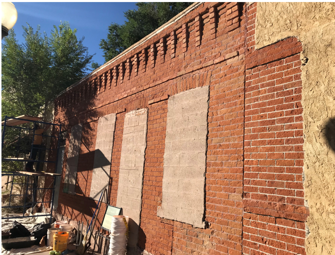
Brick Photo 4: Brick details in process of being replaced/repaiored.
