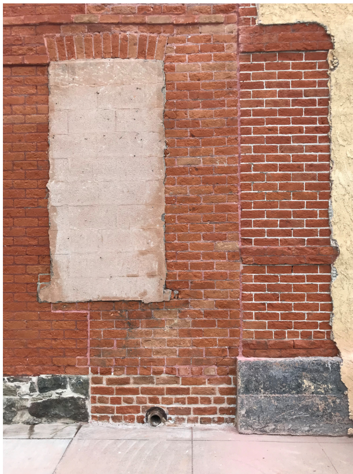
Photo 6: Note the in-filled 4' wide area that once separated the two buildings.
