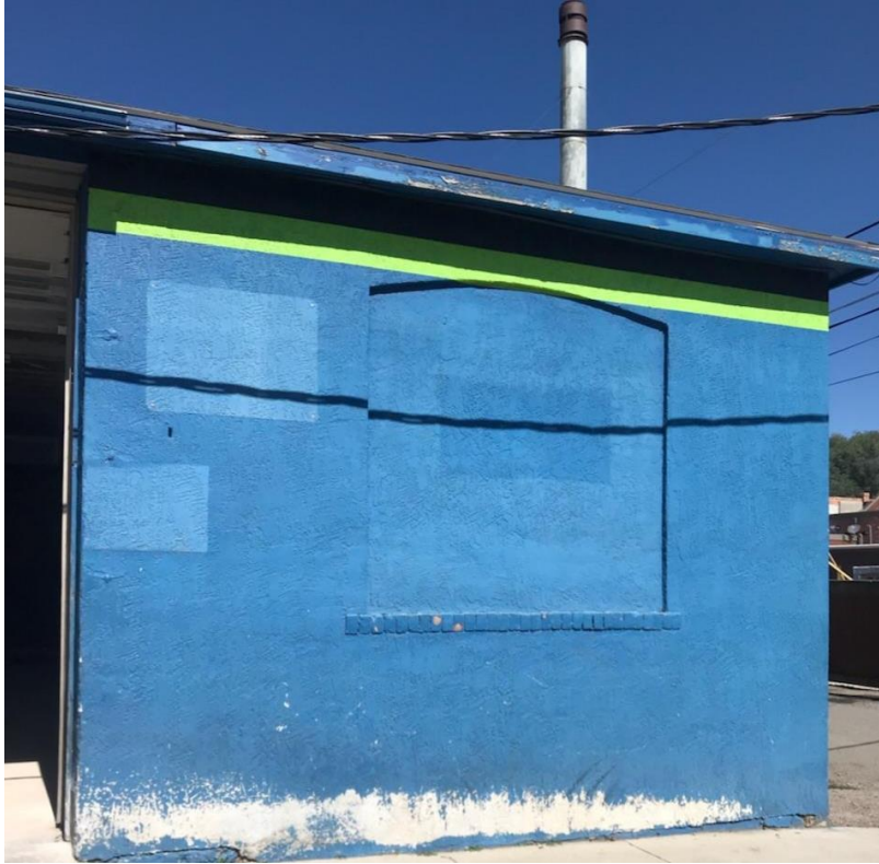
Image #6 (below), In-filled window at corner of 'E' Street and Alley, expose and replace
