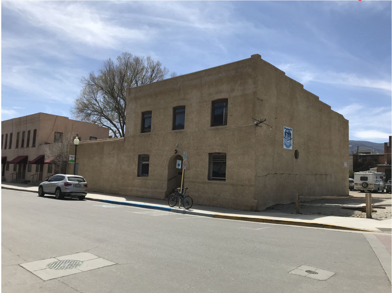
Image #1: Existing condition of Laura Evans Building (129 W. Sackett).
