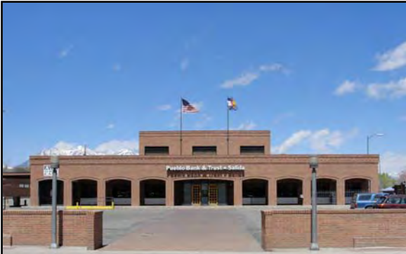
200 F St, Pueblo Bank & Trust – This building is incompatible with the character of the surrounding historic district.
