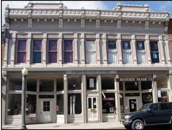
131-33 E. First St, Williams Grocery – This 50' wide historic structure utilizes breaks in the lower façade to create separate modules.
