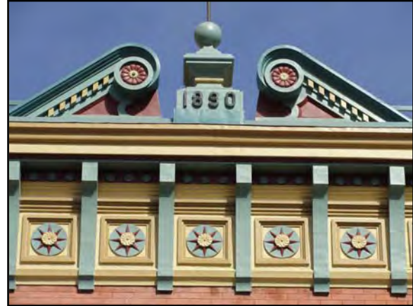
126-32 F St, Hively Block – The cornice provides a strong termination of the facade.
