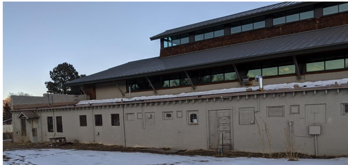
Exterior of Salida Hot Springs Aquatics Center
