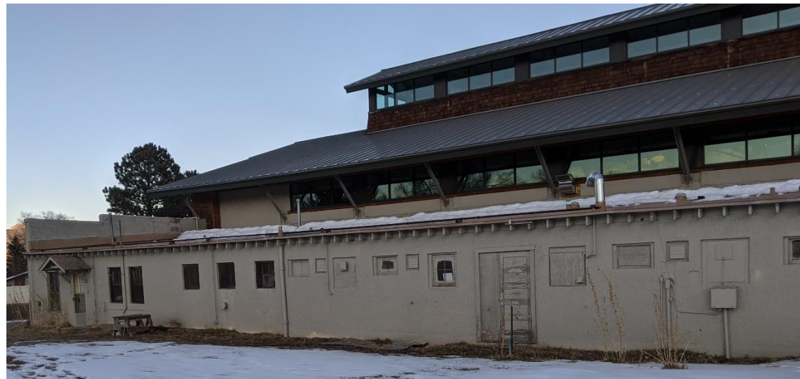
Exterior of Salida Hot Springs Aquatics Center
