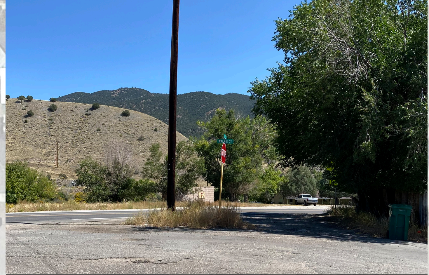
4 The intersection of CO 291 and Walnut St. will be rebuilt to replace existing open asphalt with curb and gutter, curb returns, and pedestrian facilities.
