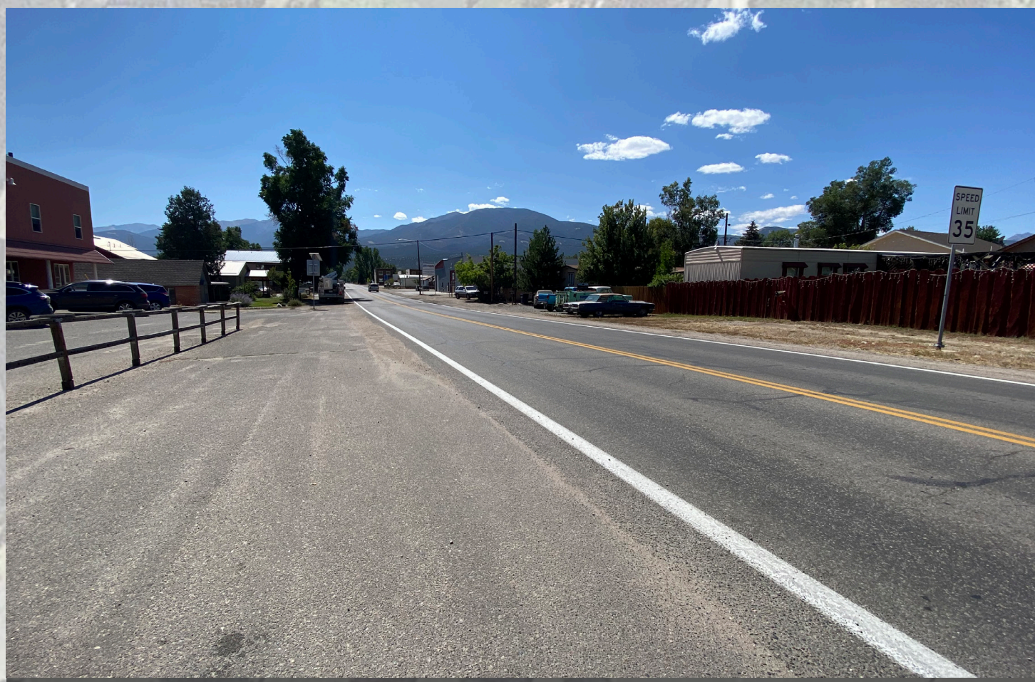
1 Existing asphalt driveways and parking areas will be sawcut for proposed widening, then replaced out to the limits of construction improvements.
